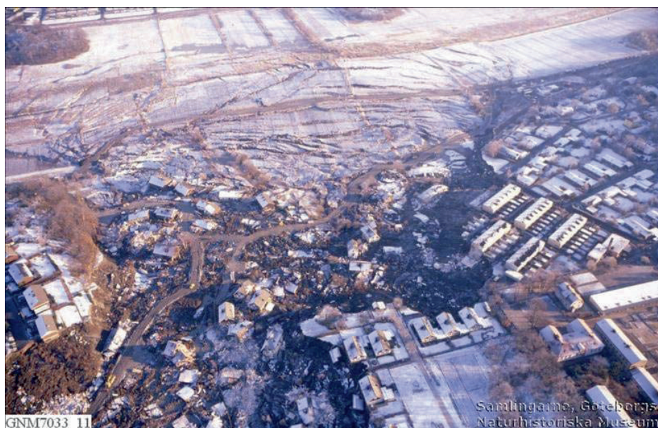
Figure 5:1.3 Aerial photograph of the Tuve slide.
